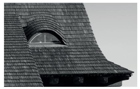
The simplest form of wood shingle is a rectangle about 16 inches (41 cm) long. The sides and butt of a shingle are often irregular; the sides may taper and the butt may not be square with the sides. Shingles that have been processed so that the butt is square to the sides are called rebutted and re-squared or rebutted and re-jointed shingles, often abbreviated as R&R.
