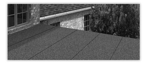
A roof that is nearly flat or slightly pitched is called a flat roof or low slope roof—no roof should be dead flat because it must have at least a slight slope to drain.
